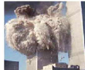
WTC 2, South Tower's destruction exhibits features explicable only with the use of powerful explosives
