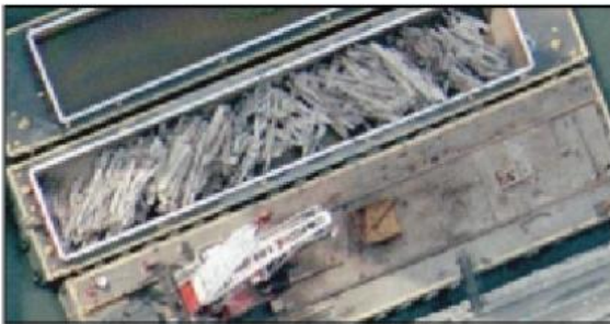
Instead of being analyzed to determine the cause of failure, most of the WTC steel was rapidly shipped off to China for recycling.
