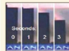
WTC 7 free-fall through 40,000 tons of structural steel designed 5x stronger than necessary - in just 4.5 seconds
